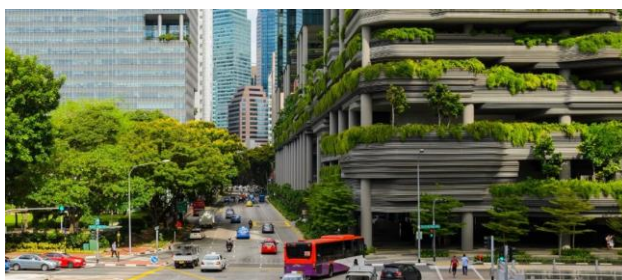
Photo: Vertical greenery attached to a building in Singapore.
